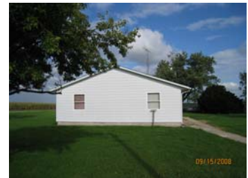
West side of house
