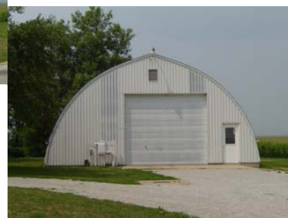
40 x 36 Shop Heated & insulated, 3 phase power
